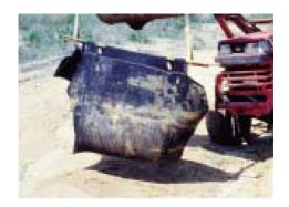
7. Move filled DrainGuard to dumping area and place on the ground
