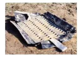
Install DrainGuard in catch basin, making sure emptying straps are laid flat, outside the basin and held in place by drain orate
