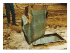
6. Remove DrainGuard from catch basin by attaching to both bars and lifting with available equipment
