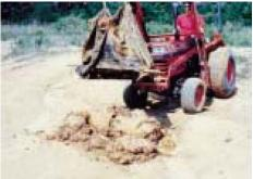
9. Lift DrainGuard by emptying straps, which are attached to the bottom of the bag. When raised by the straps, bag will turn inside-out and empty
