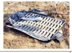
2. Hold down removal flap pockets and emptying straps by covering with soil
