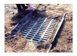
4. To prepare for emptying DrainGuard, remove soil covering removal flap pockets and insert rebar through pockets
