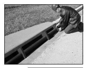
1. Place one **Anchoring Wedge** on the ends of each 3 foot section.
