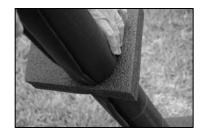
4. Align the CurbGuard Plus with the **Sediment Flap** facing down (to touch the pavement). This will form a barrier against water flowing underneath the unit and will prevent water/sediment bypass.
